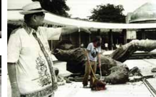
26 August 1975, Tunku Abdul Rahman inspecting damage caused by an explosion at the National Monument. The explosion was blamed on Communist insurgents.
